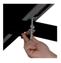
Use two nuts to secure the mounting plate to the bolts.
